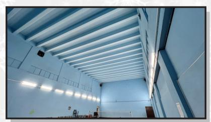
With the latest anti-glare fittings from Havells, we now have between 400 and 450 lux in the centre, which is on par with the best available lighting, that too with no glare which makes sighting easy on the eyes.
